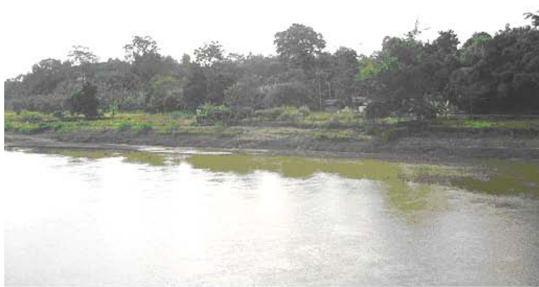
Fig. 6. The neotectonic fault scarp on the left bank of the Dhansiri River.
